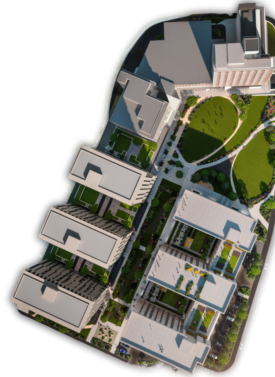
Build to Rent
