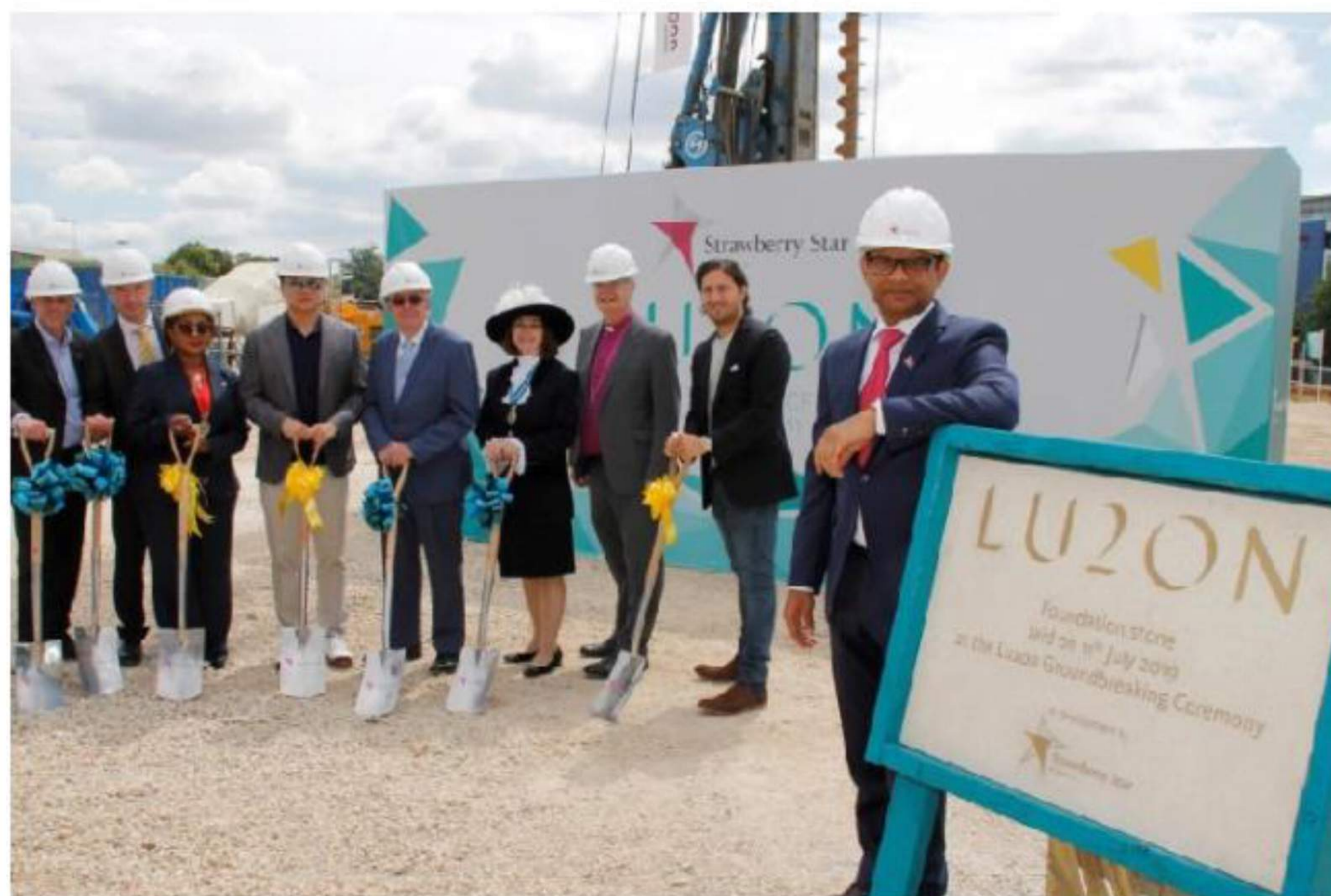
Groundbreaking ceremony as work starts on Strawberry Star Homes development in Luton
